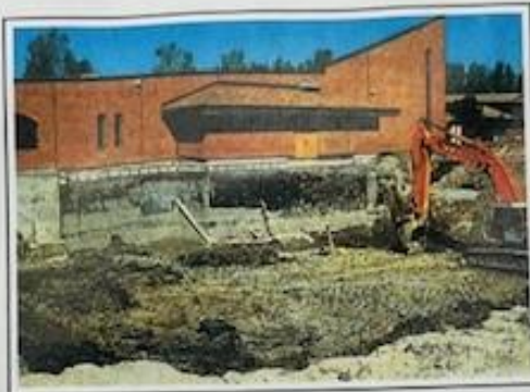
Excavating for the new Parish office and meeting rooms
